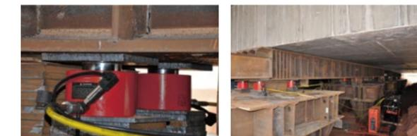
BELIUM low height cylinder used for lifting bridge
